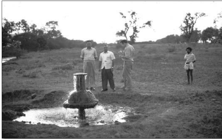
Land subsidence marked by height of top of well-casing grout above land surface, caused by underestimated rates of required pumping for mine dewatering (photos by J. Toth).
